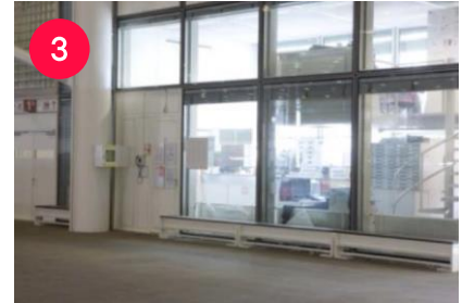
Hall 1.0, Hall manager office
