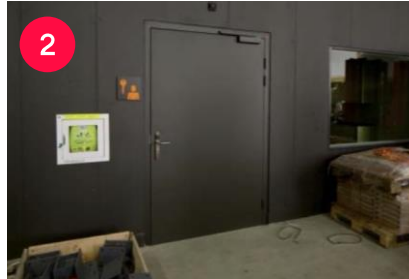
Hall 1.2, Hall manager office
