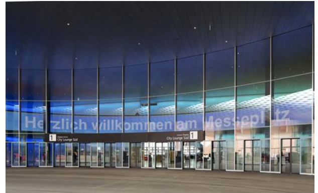
Position: City Lounge Foyer South
